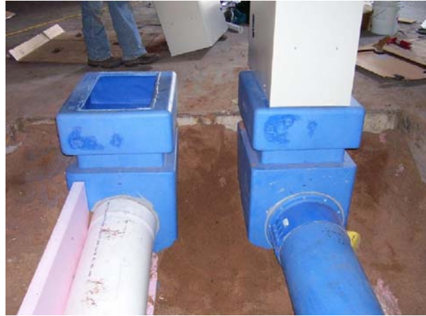
Duct and furnace attachment to the plenums
